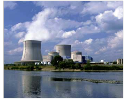
Utilities such as nuclear power plants are vulnerable to electronic and mechanical obsolescence as they are both unique and complex with life expectancies of up to 40 years.
